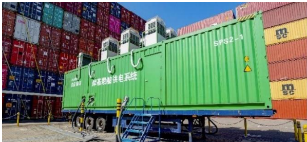
Mobile shore power system in Yantian, China. (Source: Hutchison Ports)
